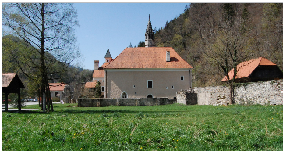
Fig. 8: Jurklošter, a view of the eastern end of the church with the former chapterhouse and sacristy (Photo: M. Oter Gorenčič)
