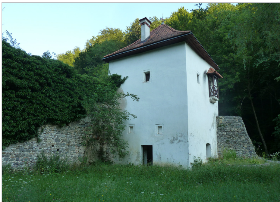
Fig. 10: Jurklošter, a part of the eastern defensive wall of the monastery complex with the Gothic tower (Photo: M. Oter Gorenčič)
